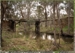
Ruins of Welsh Street Bridge
